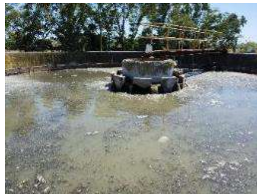
Figura 10: Tanque IMHOFF
