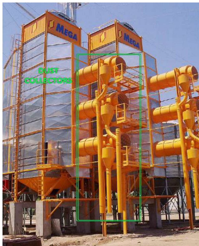
Separadores de Polvo durante montaje. Dust and Fine Collector system during the assembly process.
