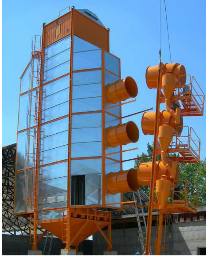
Separadores de Polvo durante montaje. Dust and Fine Collector system during the assembly process.
